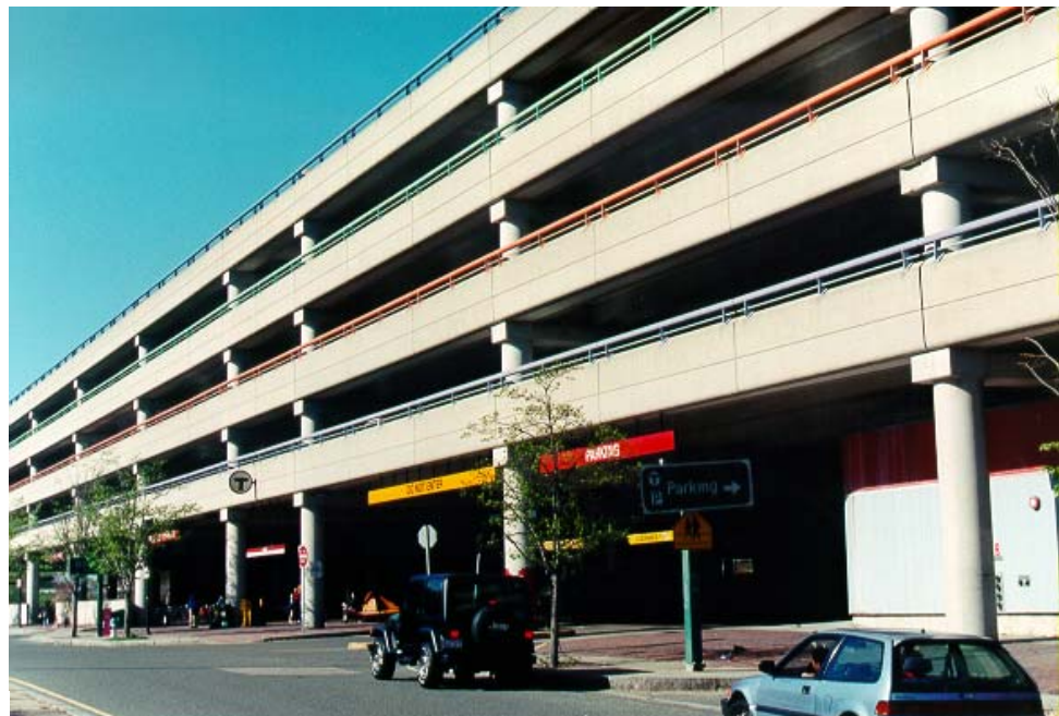
Alewife Station Parking Garage
