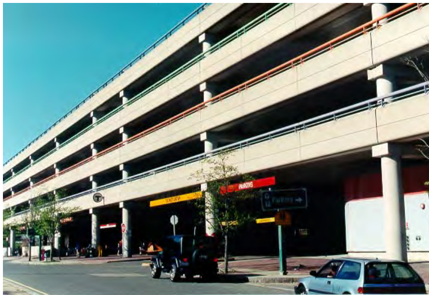
Alewife Station Parking Garage
