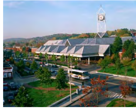
The Forest Hills Station provides service to commuter rail, bus and subway customers.
