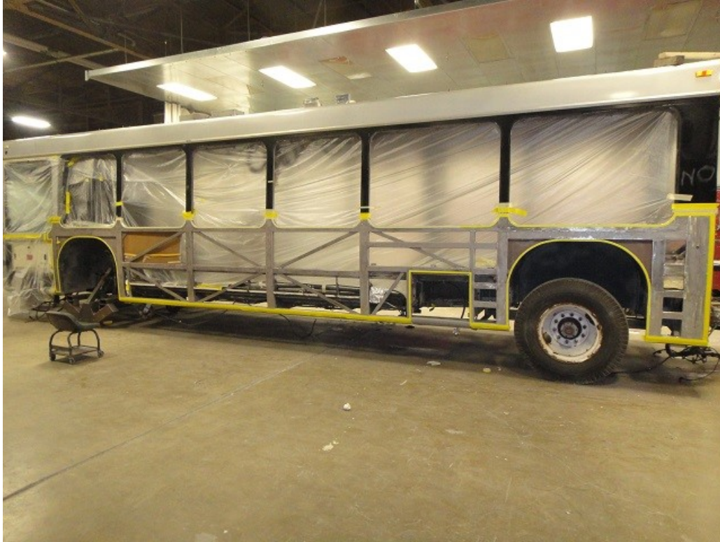
The DMA Bus Overhaul Program extended the service life of the aging bus fleet. The engine overhaul and installation of new PA44 generators, combined with various additional bus system enhancements, improved fuel economy and reduced emissions.
