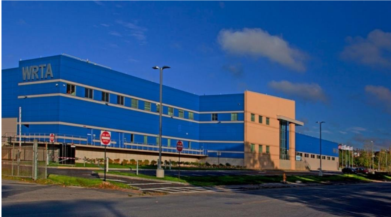
New WRTA Quinsigamond Ave Bus Maintenance Facility
