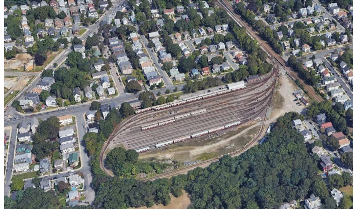
Aerial View of Existing Codman Yard (looking North)
