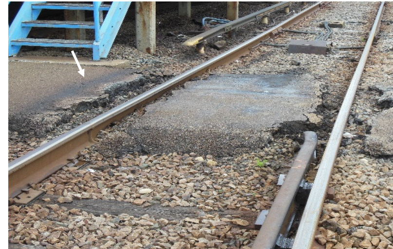
Typical Grade Crossing Condition
