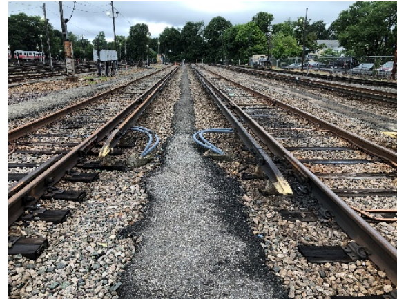
Typical Yard Conditions
