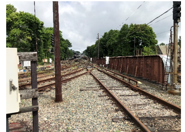
Yard Lead Tracks
