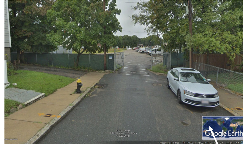
Existing Hillsdale St. Entrance
