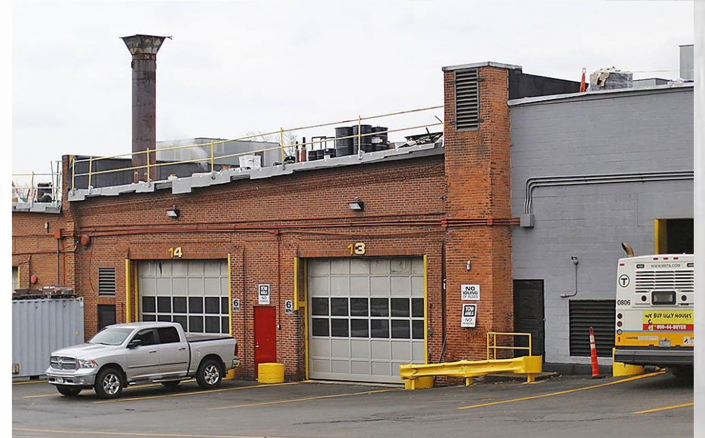
Existing MBTA garage at 954 Hancock St. Patriot Ledger photo
