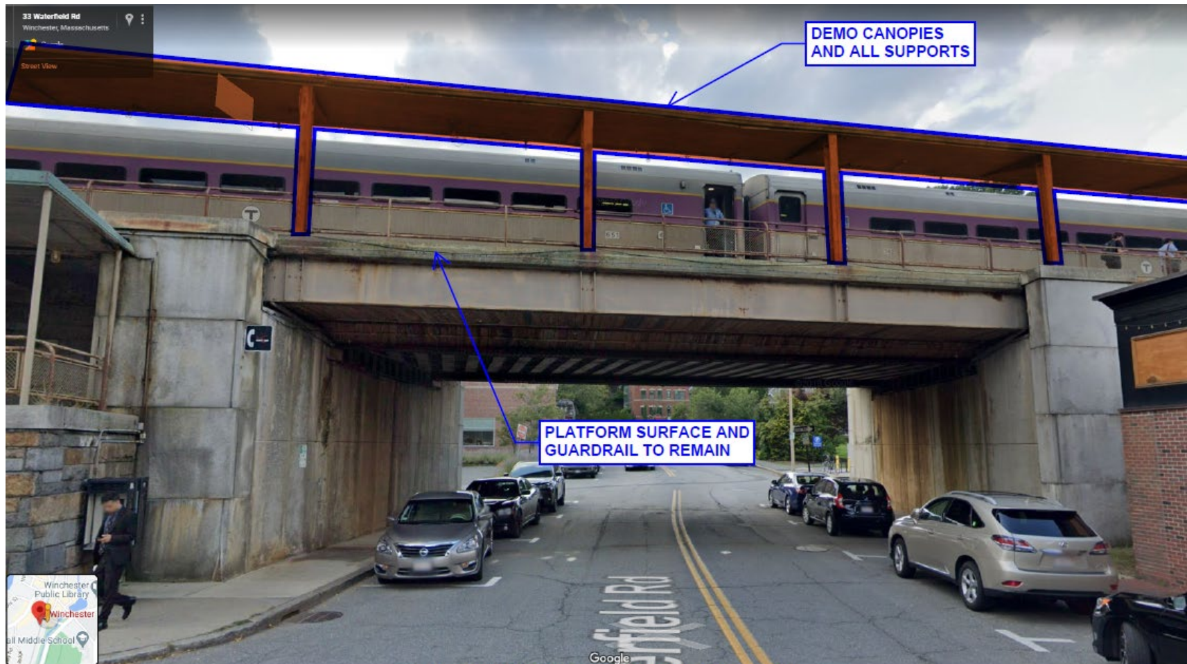
WINCHESTER CENTER STATION OUTBOUND PLATFORM / TRACK (INBOUND SIMILAR) WATERFIELD ROAD
