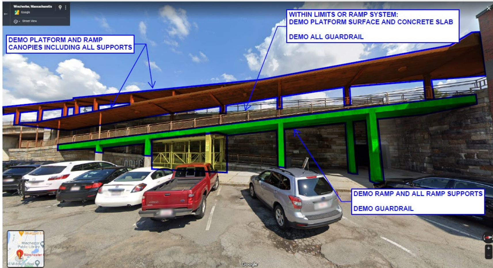
WINCHESTER CENTER STATION INBOUND PLATFORM / TRACK SOUTH END
