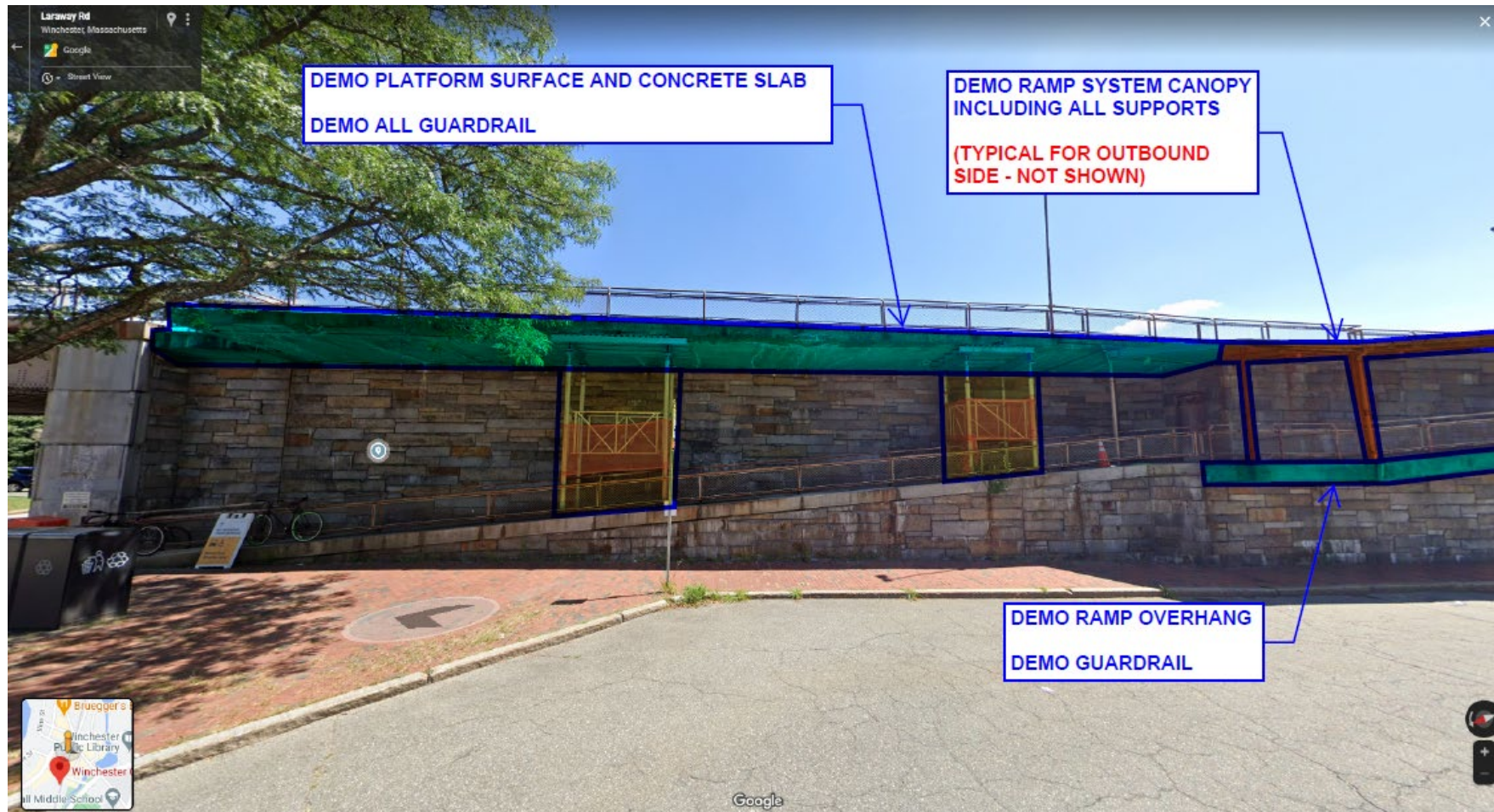
WINCHESTER CENTER STATION INBOUND PLATFORM / TRACK NORTH END
