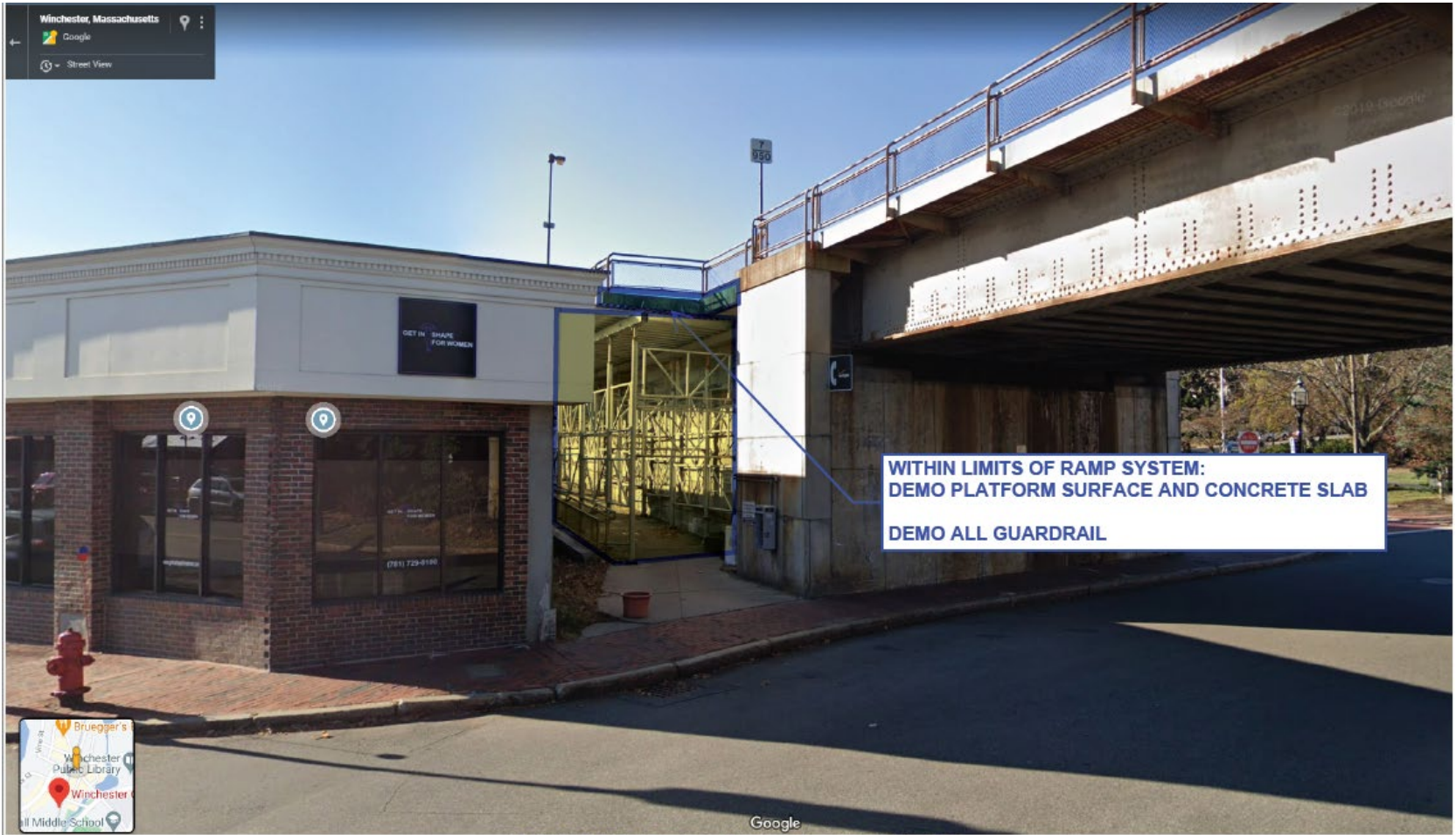
WINCHESTER CENTER STATION OUTBOUND PLATFORM / TRACK NORTH END - QUILL ROTARY
