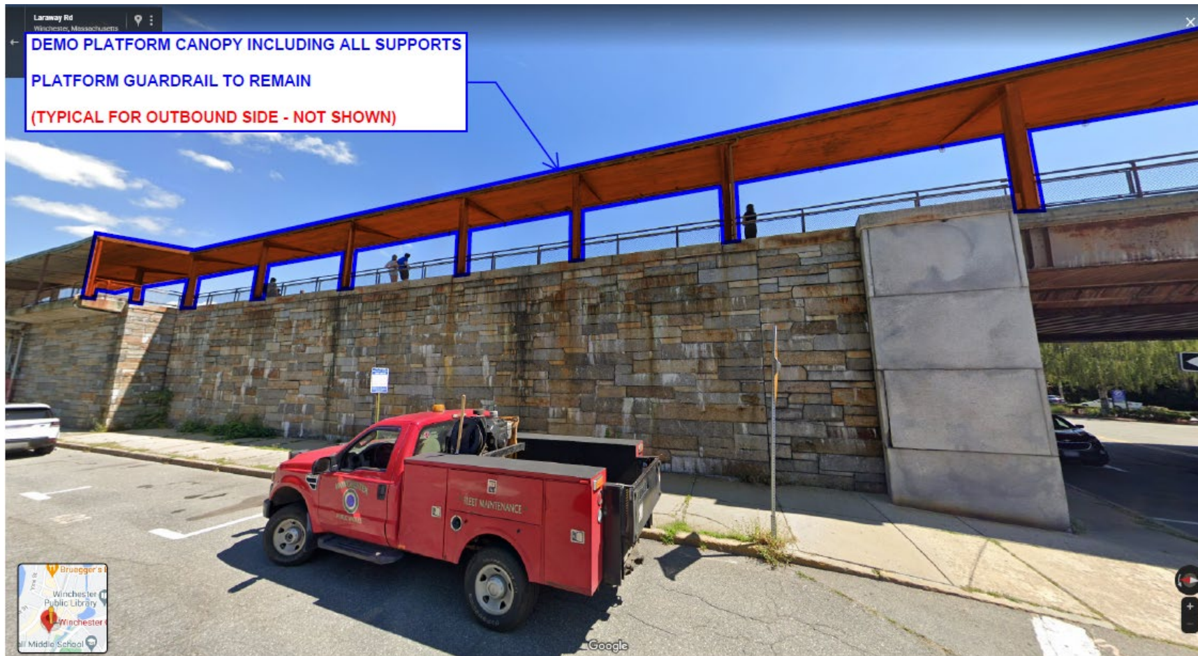
WINCHESTER CENTER STATION INBOUND PLATFORM / TRACK MIDDLE OF STATION
