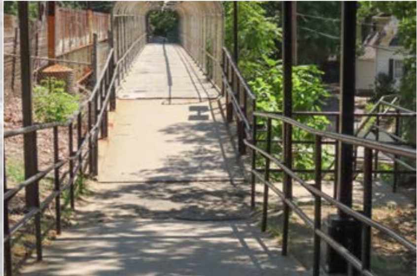
Path rebuilt to provide accessible connection to pedestrian bridge over Route 9
