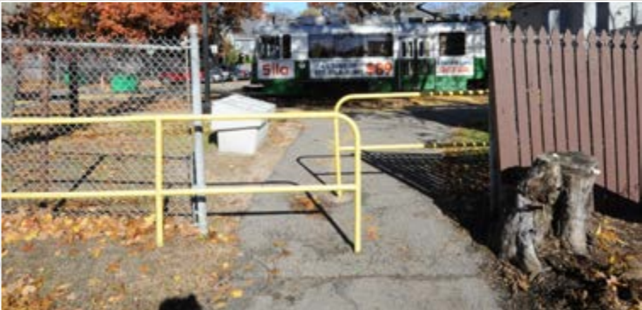
Scissor gate at entry removed
