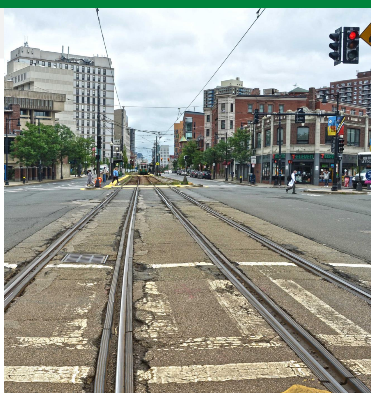
Current Conditions at Tremont St Intersection
