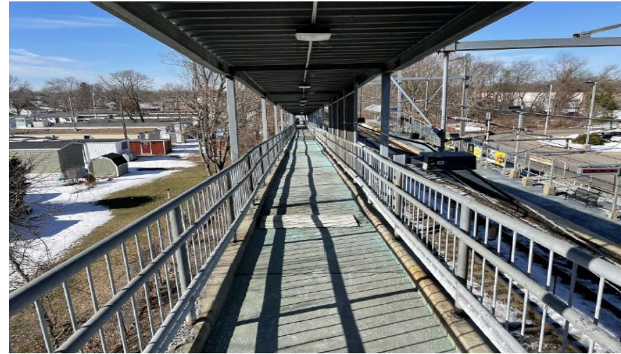
East Ramp looking West
