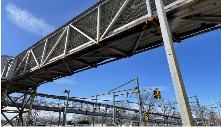
Underside of Pedestrian Bridge looking South
