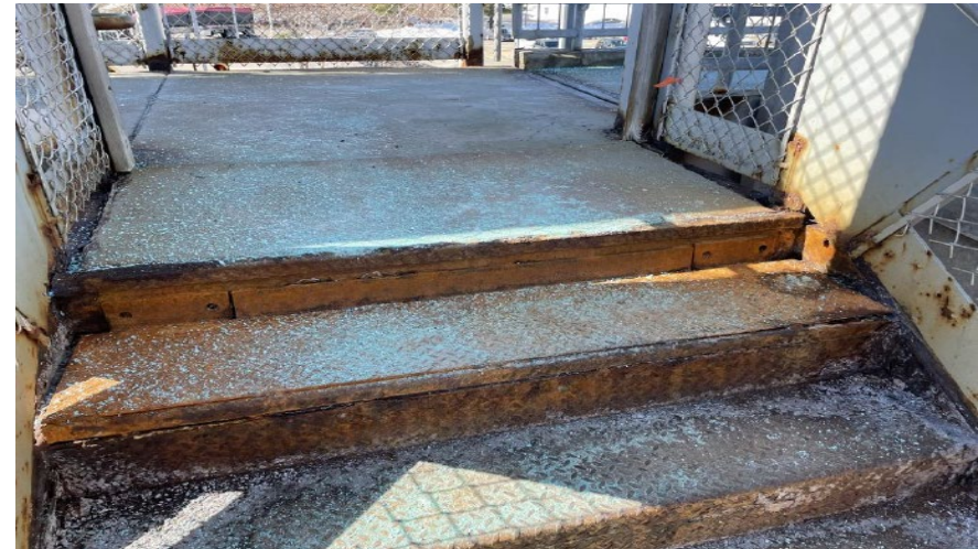
West Stairway at top landing
