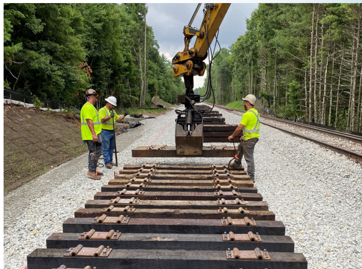
Setting ties on the right of way
