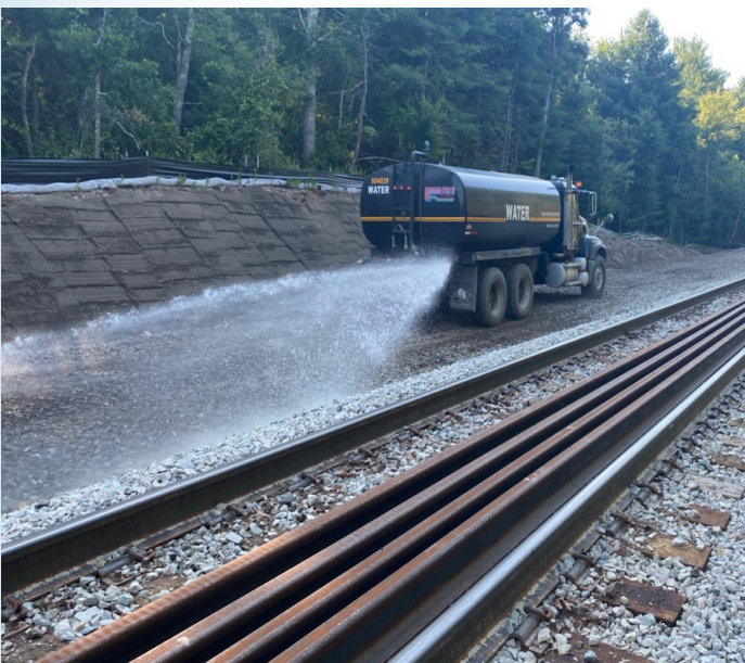
Dust control Cotley Street right of way
