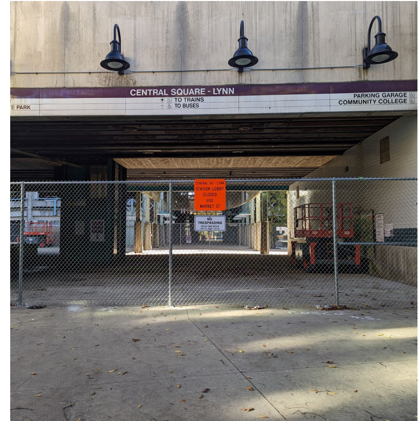
Munroe Street Fencing
