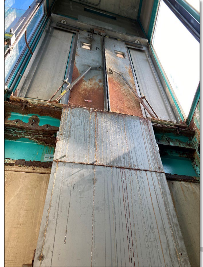
Elevator at Western Entrance near Parking Garage
