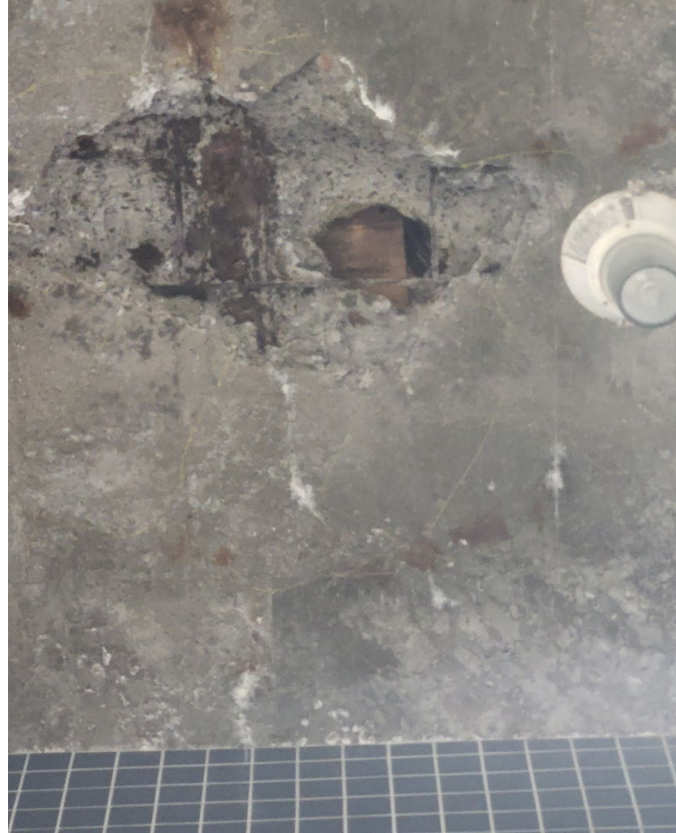
Underside of current platform
