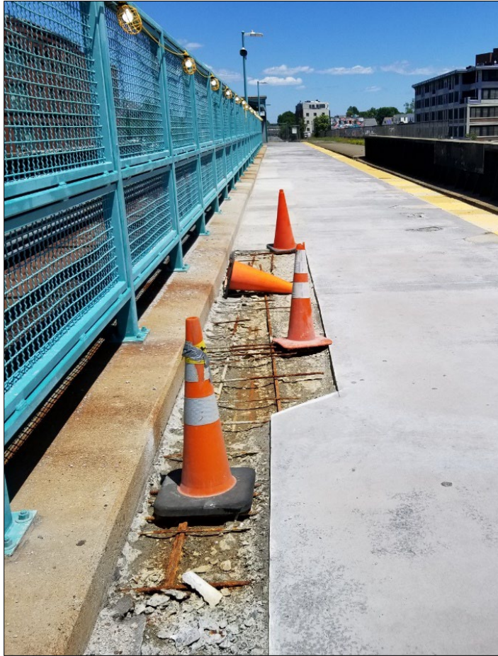
Current condition of platform
