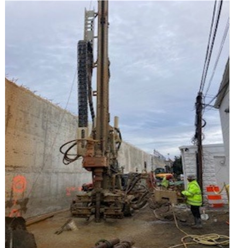
Start of Micropile Installation Work behind Thompson Street (December 2022)
