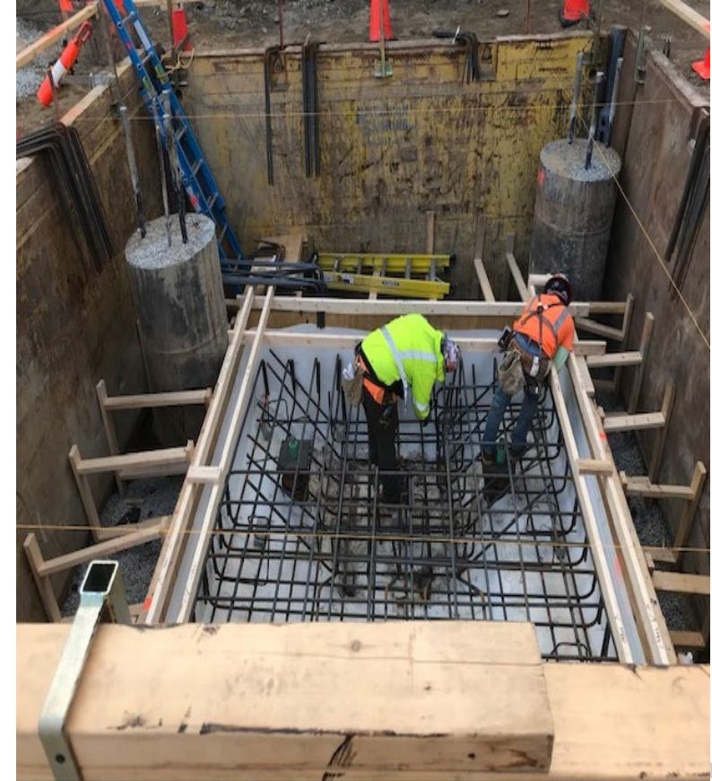
Elevator Foundation at Aberjona Lot (October 2022)
