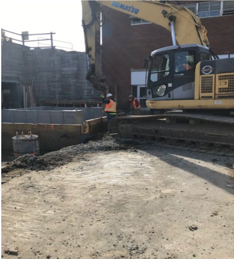
Foundation work at the Elevator Shaft at Waterfield Lot (November 2022)
