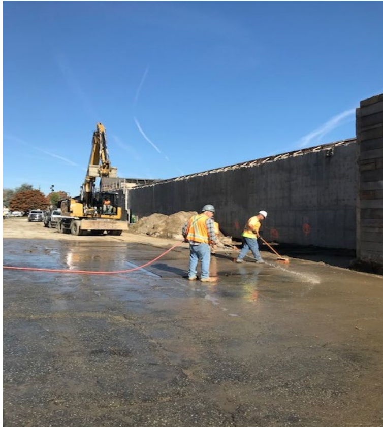
Granite Stone Removal Progress and Dust Mitigation at Laraway Road (November 2022)
