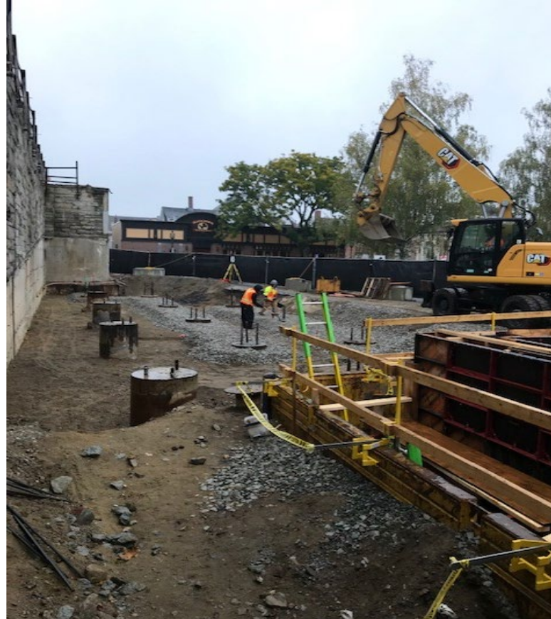
Start of Ramp Foundation at the Aberjona Lot (October 2022)
