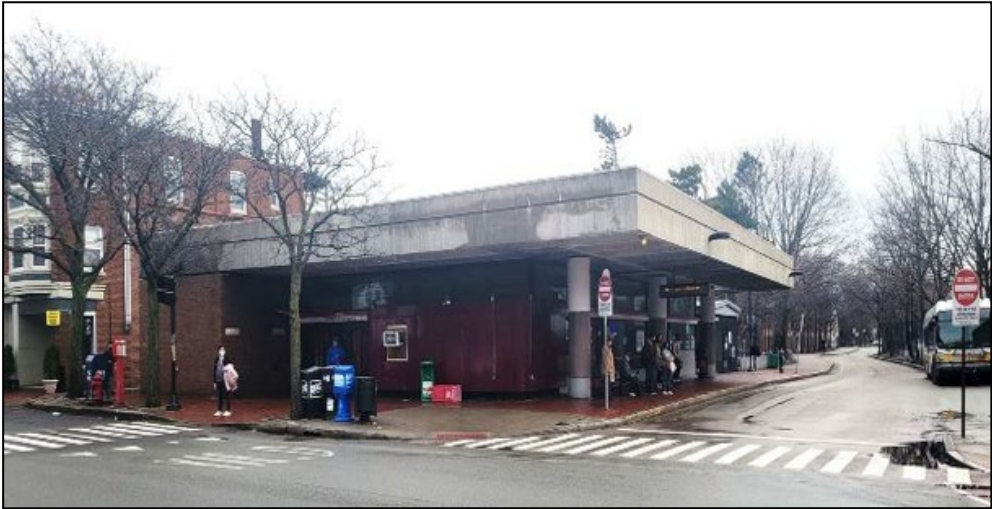
College Avenue Entrance and Bus Waiting Area
