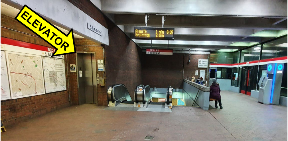
Existing College Avenue Entrance Elevator
