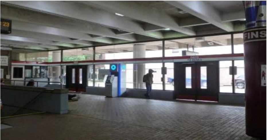
Lobby Looking Out to Bus Waiting Area
