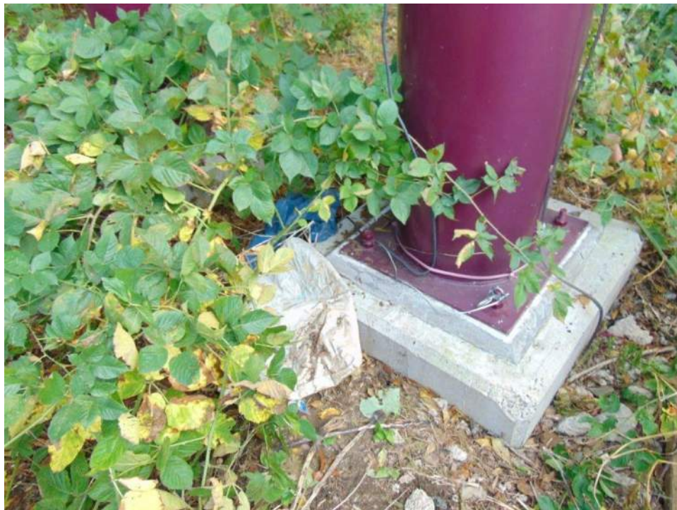
Photo 8. Data logger and reference electrode location. Pier 23
