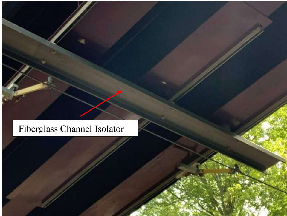
Photo 1. Catenary cable under the FRP isolation.
