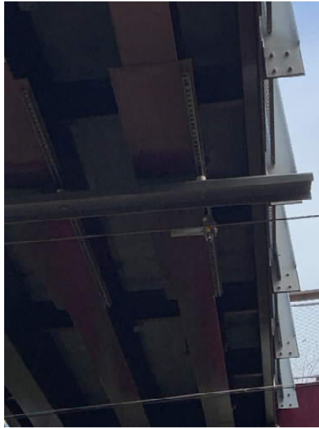
Underside of Bridge and the Catenary "shield"
