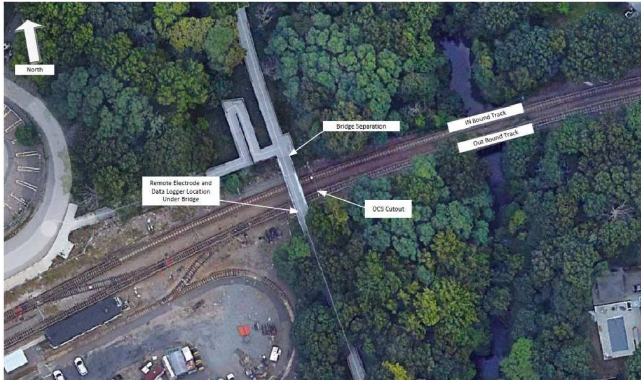
Figure 1. Aerial view of Mattapan Bridge
