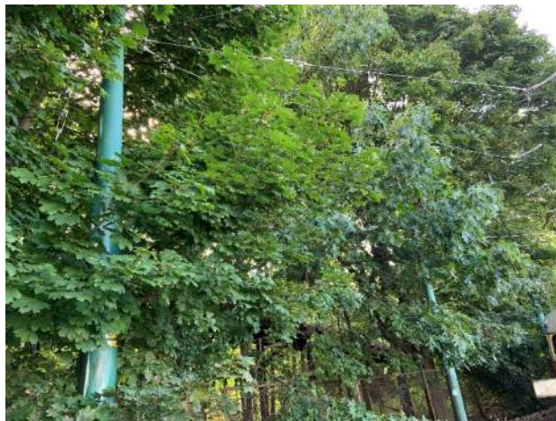
(Maintenance Loop – Tree Trimming needed)
