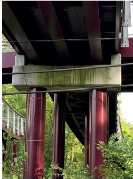
Bridge Pier 24 Looking towards Mattapan
