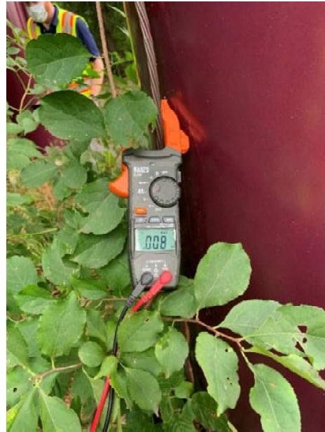
Bare Conductor (Bridge Pier 23) Measurement
