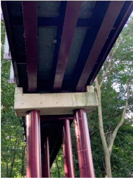
Bridge Pier 23 Looking towards Milton
