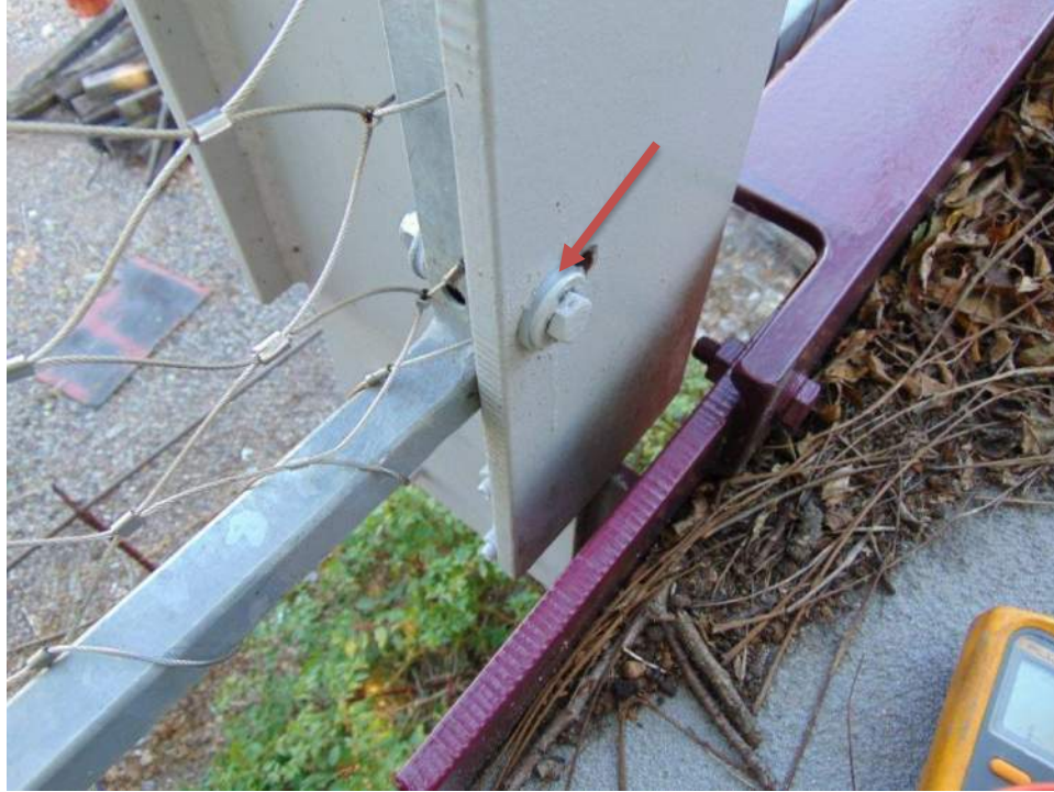
Photo 5. Isolating washer.
