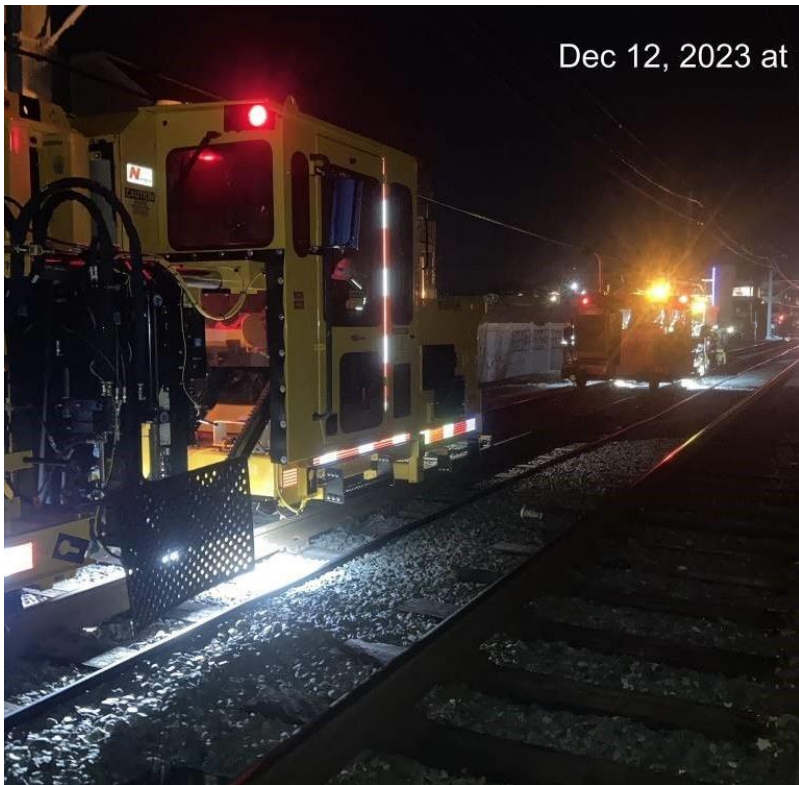
GLXC construction equipment used to re-gauging
