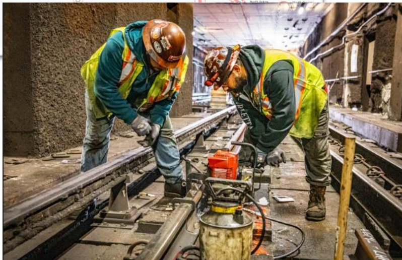
Track work on the Red Line
