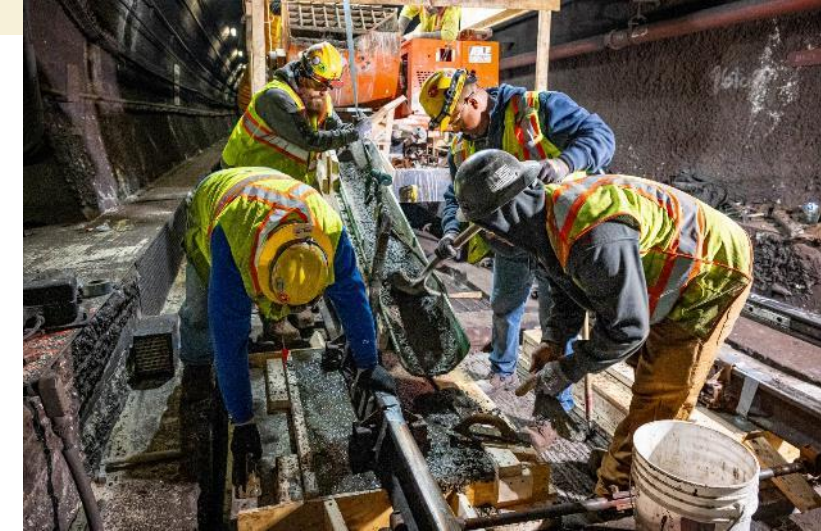
Repairing concrete slabs
