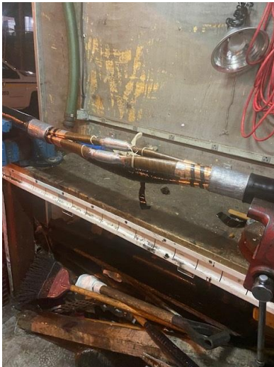
Typical Lead Splice (cable/phase connections)
