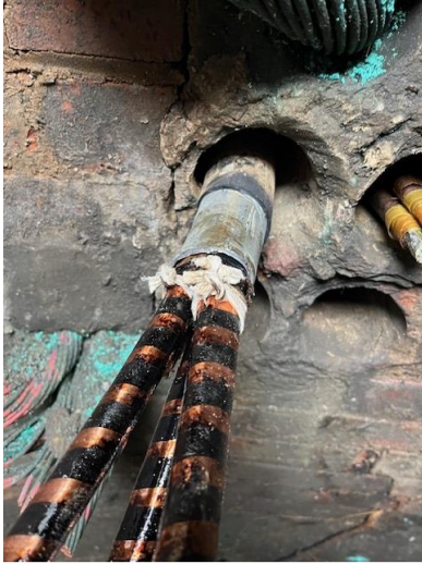
Typical Lead Splice (cable/phase connections)
