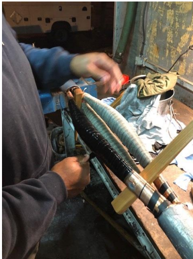
Typical Lead Splice (phase isolation & insulation)
