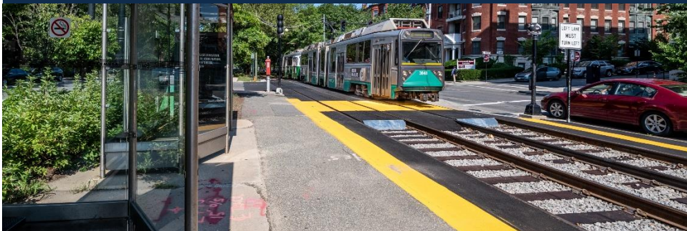
Upgraded accessible grade crossing on the Green Line's C Branch.
