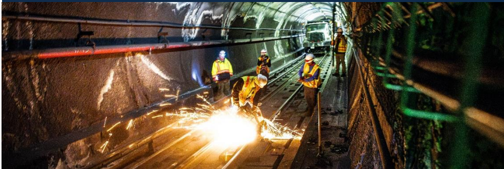
Track work during Red Line diversion as part of the Track Improvement Program.
