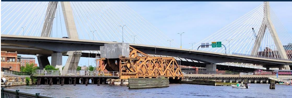
Existing 1930's North Station Draw 1 Bridge.
