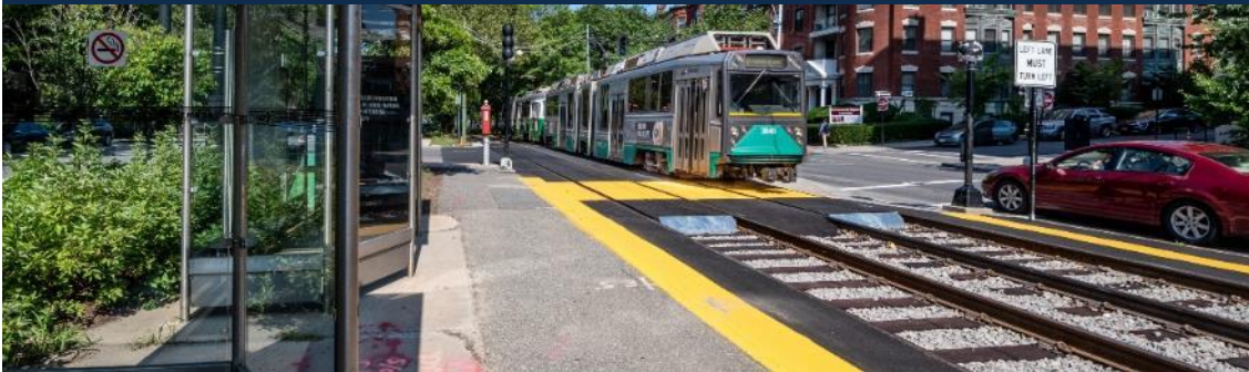
Upgraded accessible grade crossing on the Green Line's C Branch.
