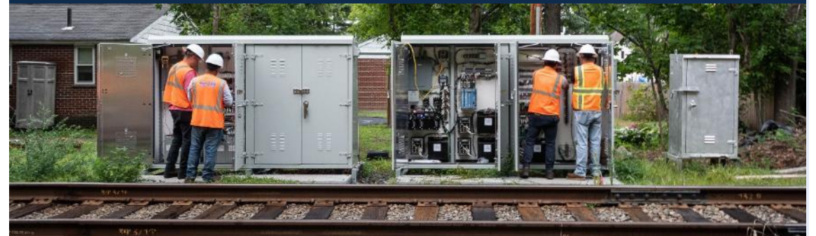
Maintenance-of-way crew performing work at our ROW.
