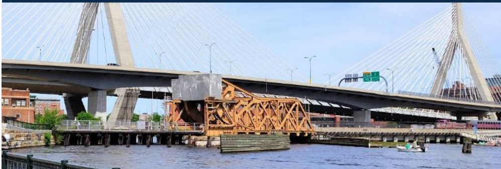
Existing 1930's North Station Draw 1 Bridge.
