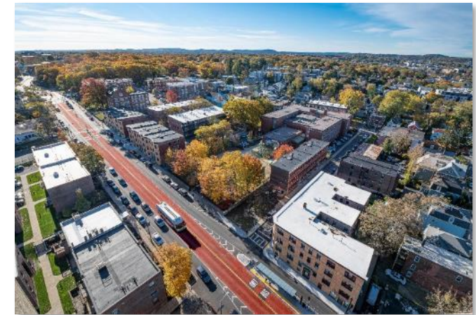
An aerial view of the Columbus Avenue bus lanes
