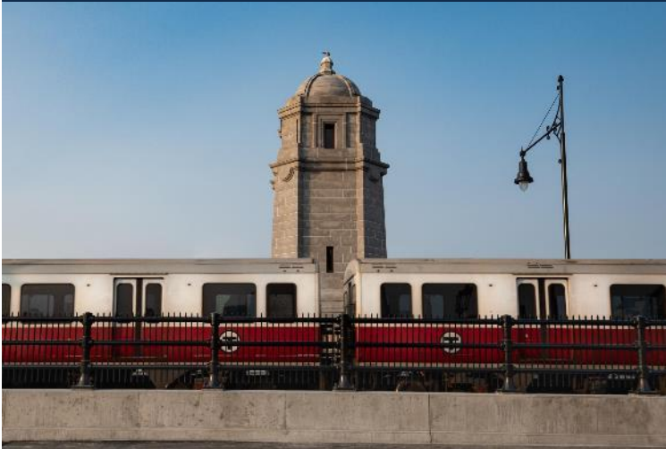
Red Line train passing over Longfellow Bridge
