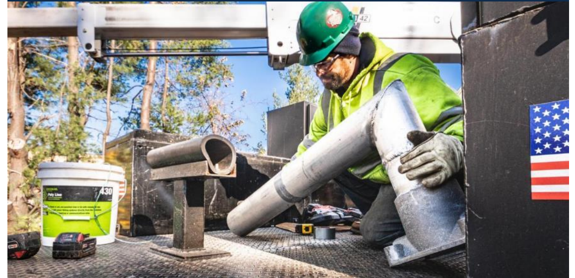
Work on signal upgrades at Kendal Green Station in Weston, MA
