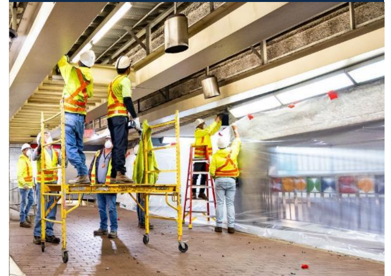
Ceiling work in progress at Andrew Square Station
