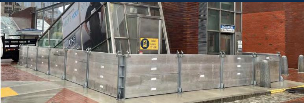
Flood plank deployment for flood mitigation at Aquarium Station.
