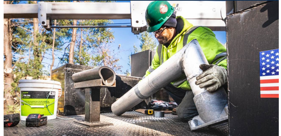
Work on signal upgrades at Kendal Green Station in Weston, MA
