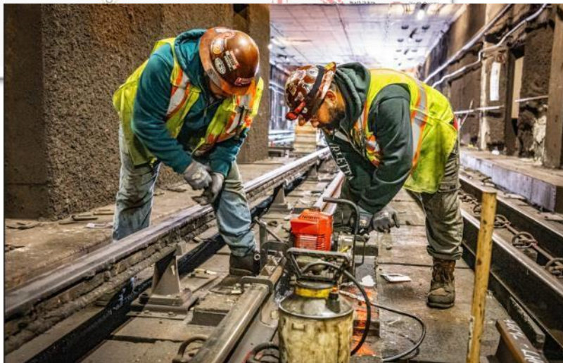
Track work on the Red Line
