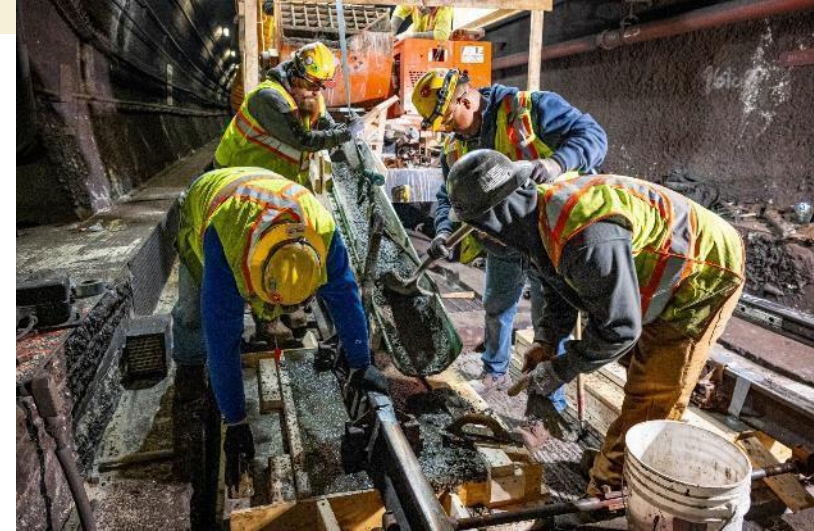
Repairing concrete slabs
