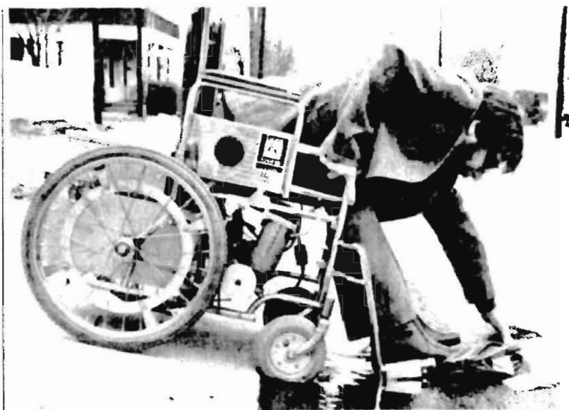
Lip on Curb Cut
