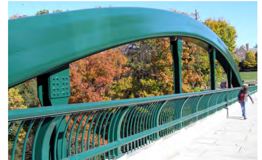
Thurston Avenue Bridge Ithica, NY
