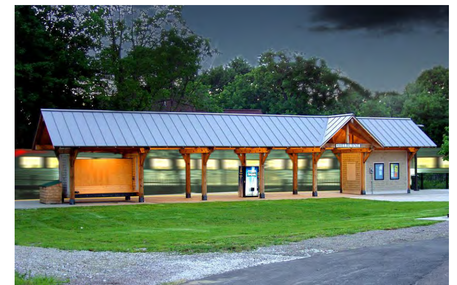
Shelburne Station Shelburne, VT
