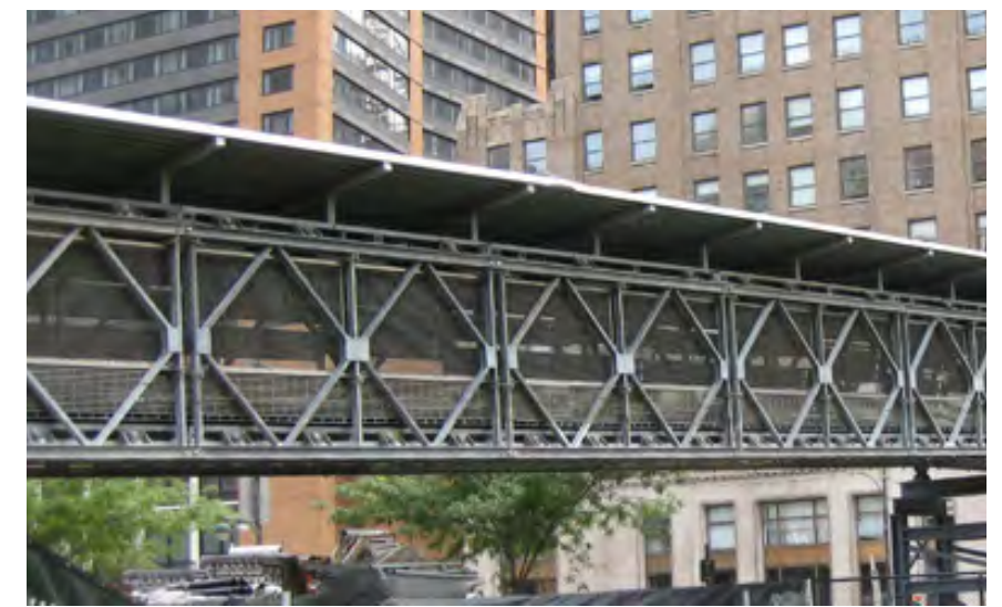
Pedestrian Bridge over Highway New York, NY
