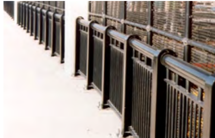
Broadway Bridge Boston, MA
