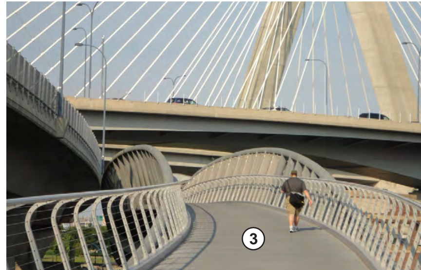
Steel and FRP Pedestrian Bridge Cambridge, MA
