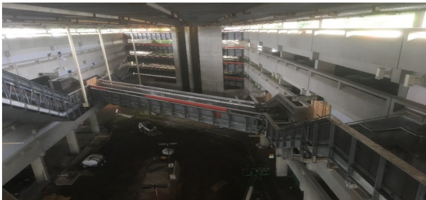
Quincy Adams Roof Platform & Staircase Demo
