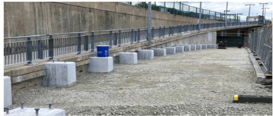
Braintree CR Canopy Foundations/Columns
