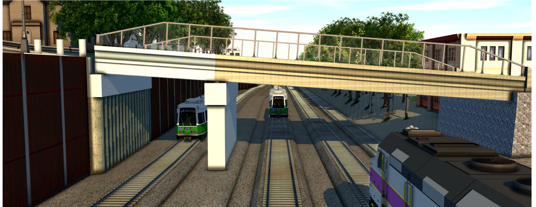
Figure A5.2.2-10: An east elevation (looking west) showing the Medford Branch Westbound rail line passing below the new additional span of the School Street Bridge. The existing superstructure (darker concrete) remains along with the existing granite north abutment, the new span (lighter concrete) is supported by a secant pile wall abutment on the south side, and a wall pier that will support the new span and the south side of the existing superstructure. Bollards for the Community Path are shown behind and above the secant pile wall abutment, which will act as barriers for the path.
