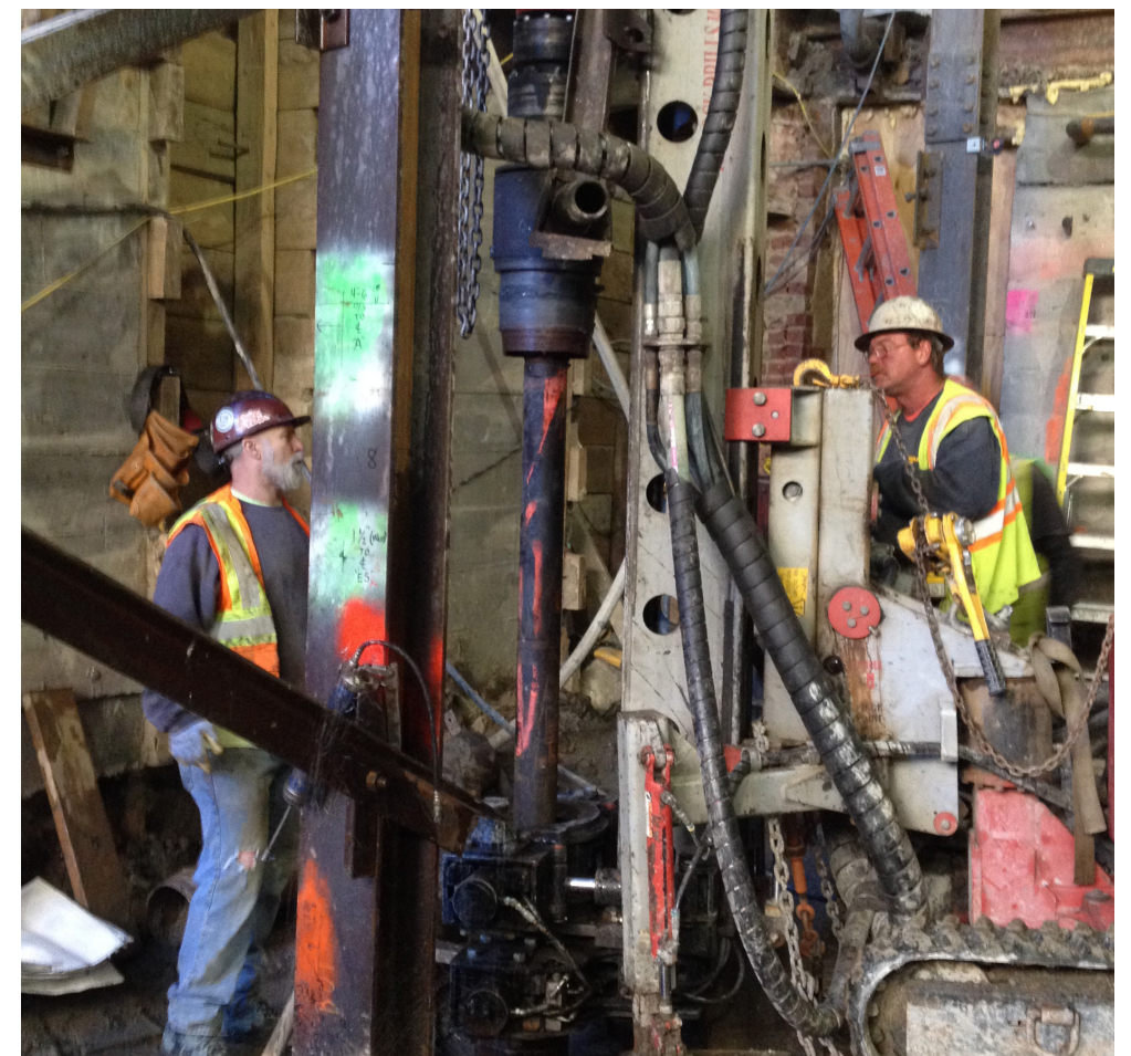
Figure A5.2.2-7: In designing for restricted access in busy urban environments similar to the GLX project alignment, GLP has incorporated micro-pile walls in restricted access similar to the ones seen here from New York's Second Avenue Subway Project.
