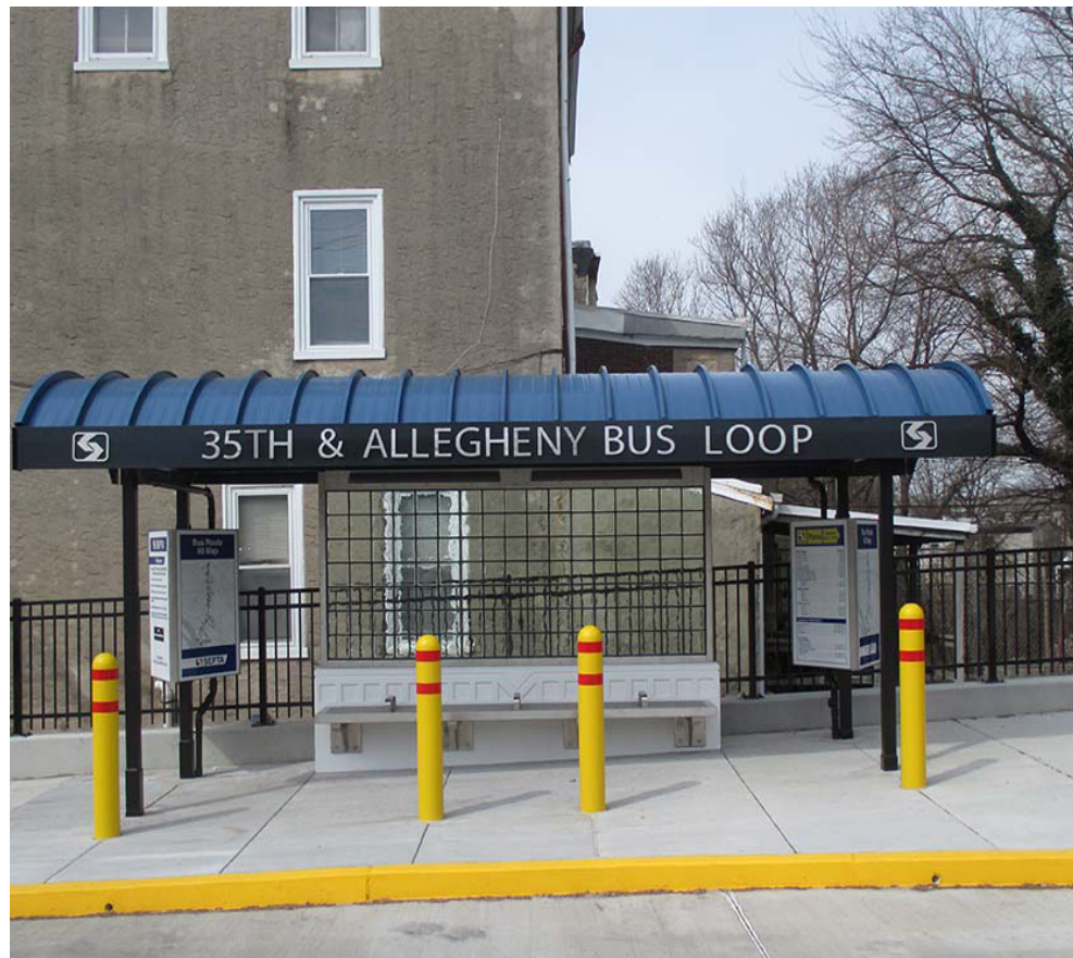
Figure A5.2.3-5: Bus shelter and fencing at the 35th and Allegheny Bus Loop. The solid glass block and open picket fencing provides visual surveillance for passengers approaching and waiting in the shelter.
