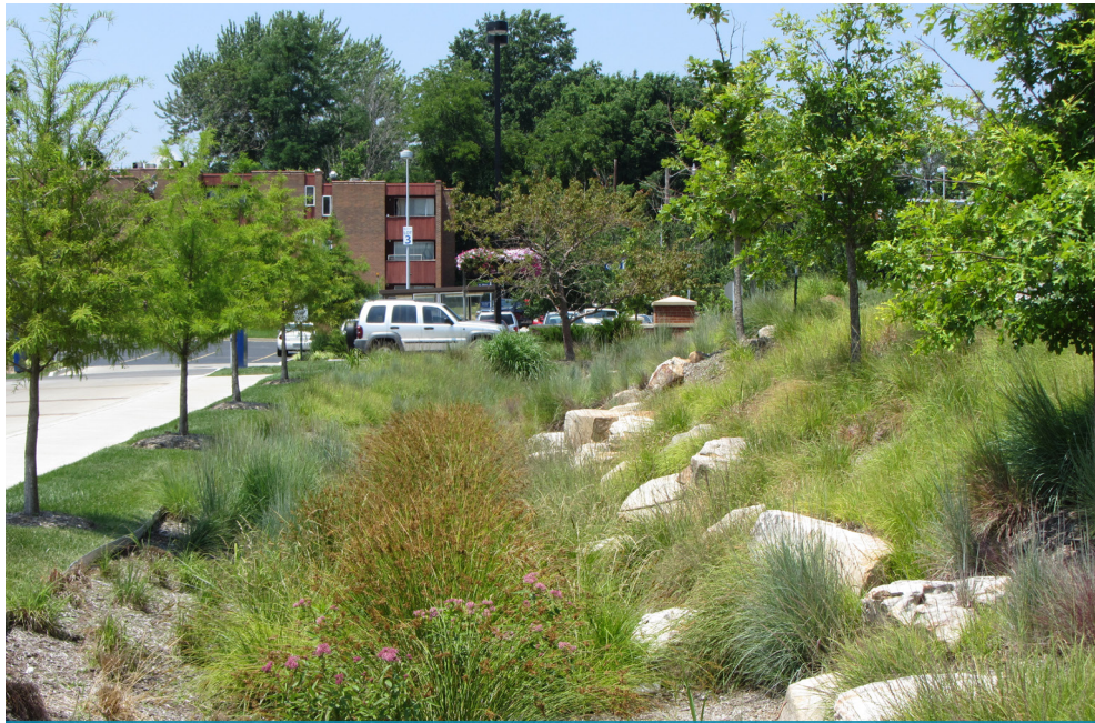
Figure A5.2.4-2: As demonstrated by the Beckley Intermodal Gateway in West Virginia, GLP designers have successfully designed slope stabilization and stormwater management plantings that use low-maintenance native plant species.
