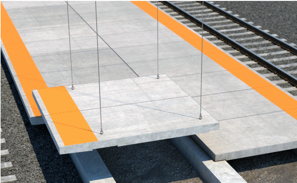
Figure A5.2.3-3: - Precast concrete platform panels with the tactile edge installed prior to delivery at the job site. This method was used on Southeastern Pennsylvania Transportation Authority (SEPTA) to provide high-quality fabrication and improve construction efficiency.
