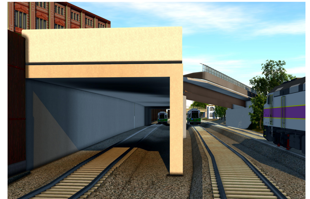
Figure A5.2.2-13: An east elevation (looking west) showing the railroad tunnel behind and against the south abutment of the Medford Street bridge carrying the Medford Branch Westbound rail line. The tunnel is composed of precast concrete arch segments supporting 5 feet of soil above, retained by the headwall shown above the tunnel.
