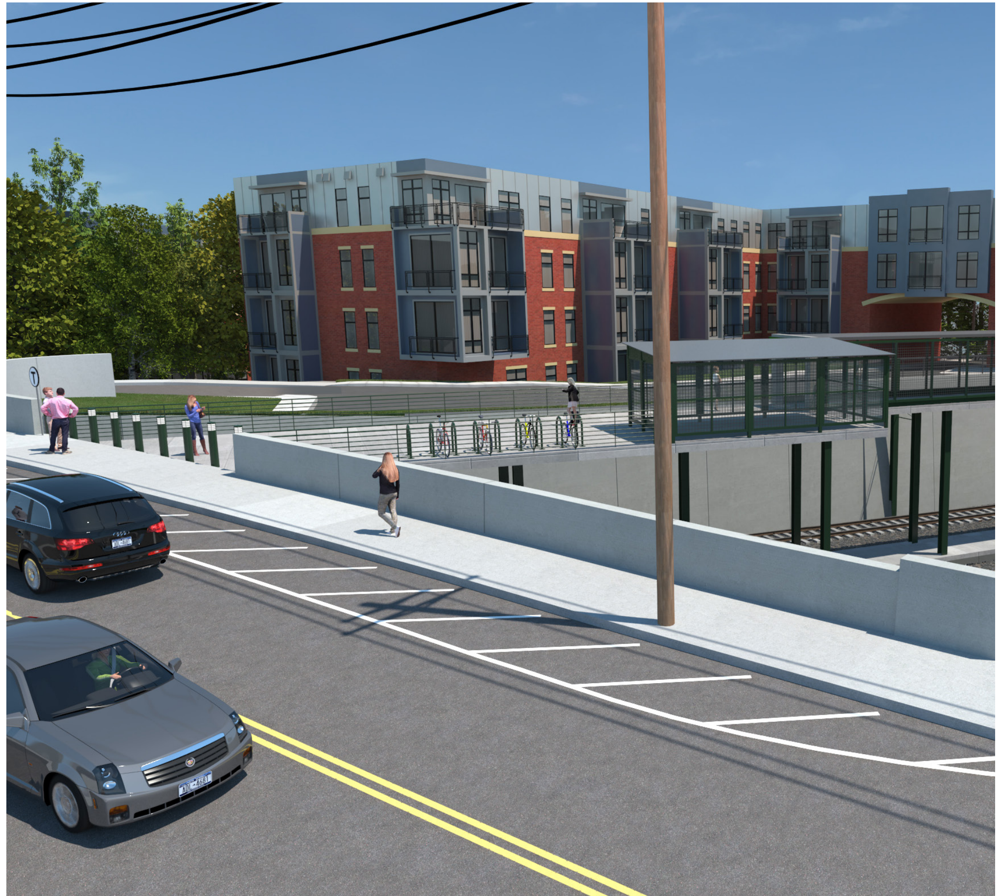
Figure A5.2.3-10: Entrance to Magoun Square Station showing bollards and the interface of the highway ROW and the station entry.
