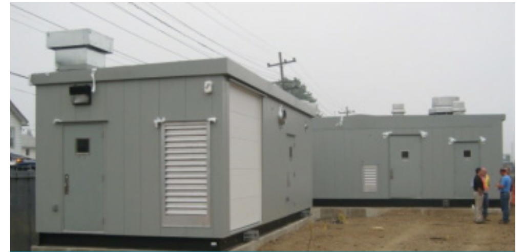
Figure A5.2.1-11: GLP’s approved Alternative Technical Concepts (ATC) offers prefabricated TPSSs that will allow MBTA to witness full functional testing in the factory, thereby eliminating unknown conditions and eliminating potential schedule impacts.
