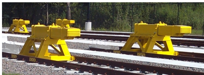
Figure 4.1-11 LRT hydraulic bumping posts located at stub-end tracks.
