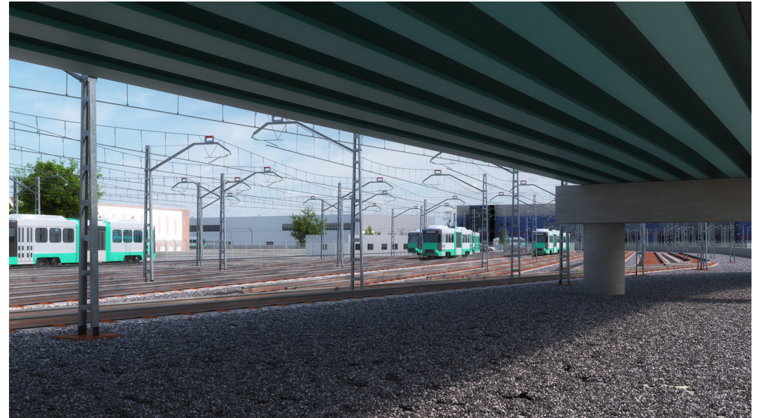
Figure 4.2-3 Viaduct over yard. View of the Union Square westbound elevated guideway (viaduct), VMF yard, and Vehicle Maintenance Building.
