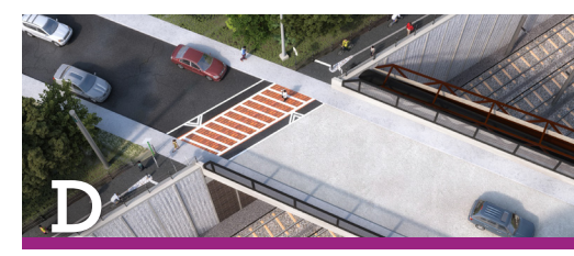
D Walnut Street Community Path. WBG optimizes the Walnut Street Community Path underpass by placing the path at street level.
