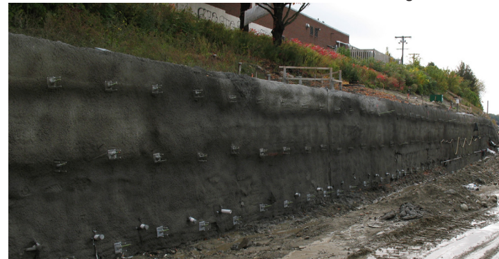
Figure 4.2-5 Soil nail walls. Soil nail walls at Jacobs' Winter Street project are similar to those that will be used at the Lowell Street Bridge.
