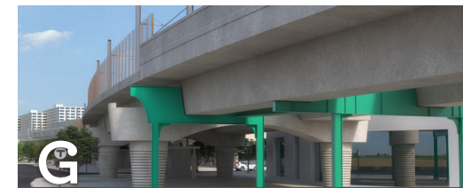
G Lechmere Viaduct. Located in East Cambridge, the double track structure will support eastbound and westbound tracks of the Medford Branch alignment.
