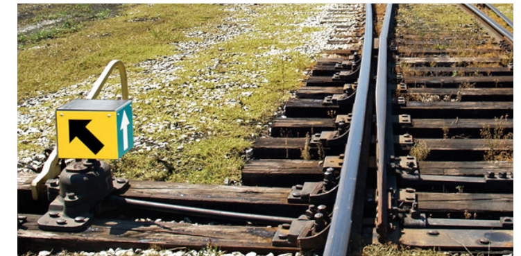
Figure 4.1-7 Hand throw switch. WBG incorporated hand throw switches with an easy-throw handle and cube direction indicator for optimal safety.
