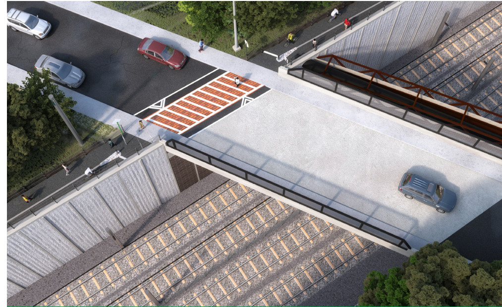
Proposed Walnut Street Bridge. WBG's ATC 2 eliminates the pedestrian underpass, improving track sight lines and increasing pedestrian safety.
