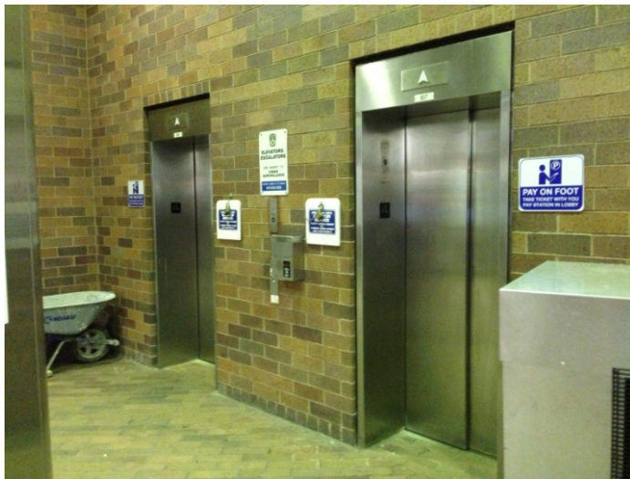
Garage Elevators 806/807 at Lobby
